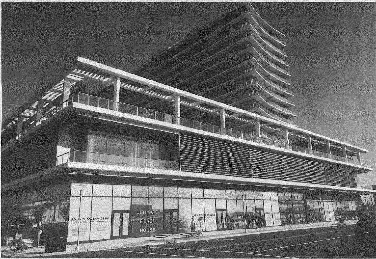
The Asbury Ocean Club is near completion
